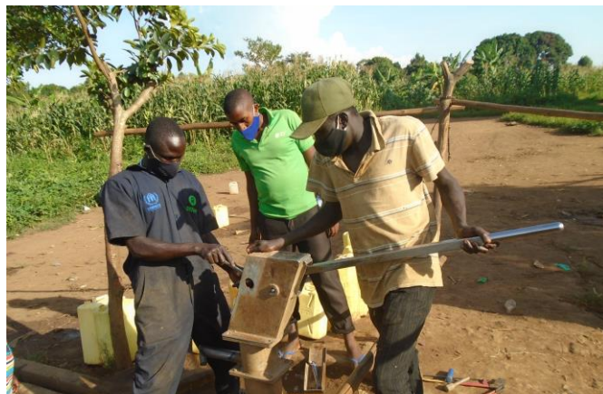
Mark (Left) repairing a broken borehole hand pump
