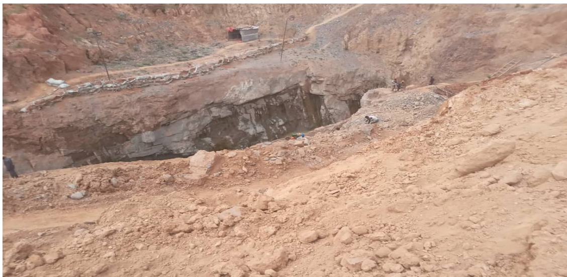
Figure 5. A deep hole created at Tiira gold mine in Busia
