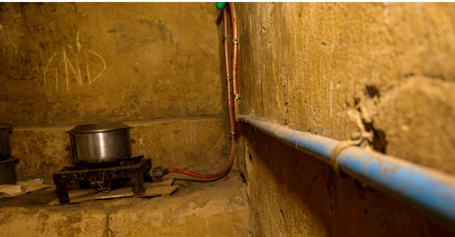
A biogas cooker connected to Albert's kitchen. ~ Photo by Derrick Kaweesi/ Oxfam
