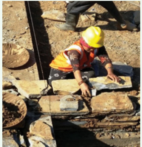
Dil Kumari working on a stone wall. Photo by: Nishant Mahat/Oxfam
