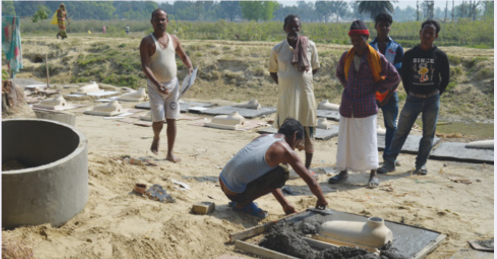
People of Mushar Community constructing toilets. Photo credit: SDRC
