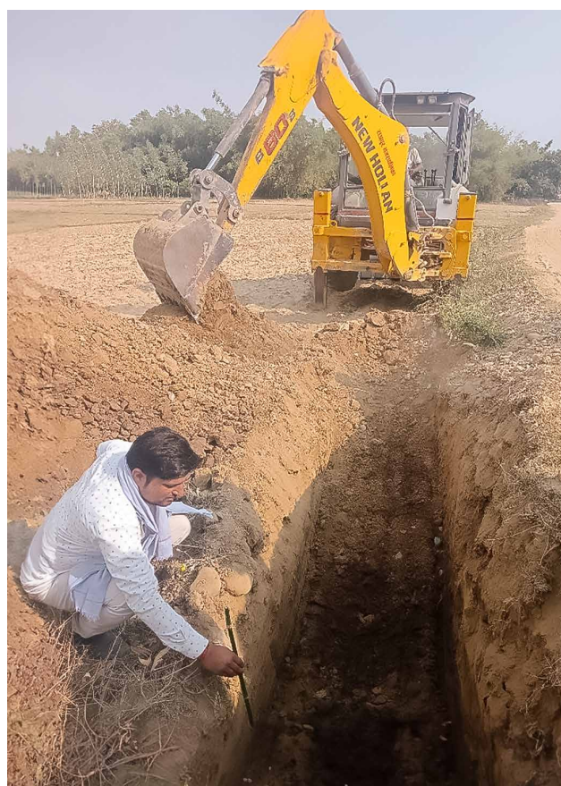
The Rajpur Water and Sanitation Board manager ensures the depth of the water main excavation. Photo: RDC Nepal, Rautahat.
