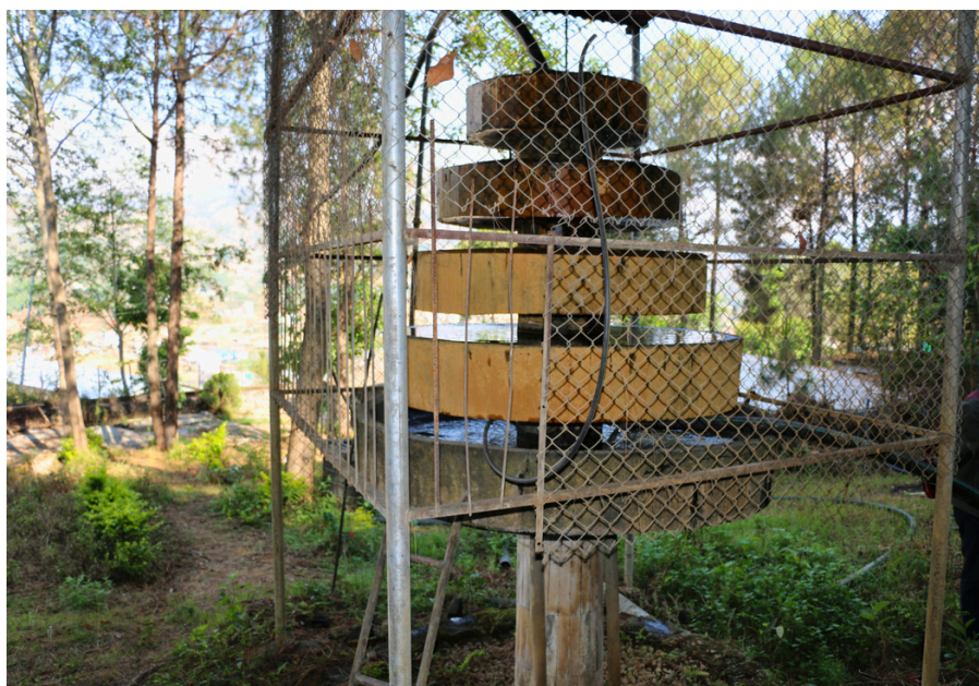
Water filtration unit constructed under Bhakundebesi WSS. Photo: Rachana Mukhia/Oxfam
