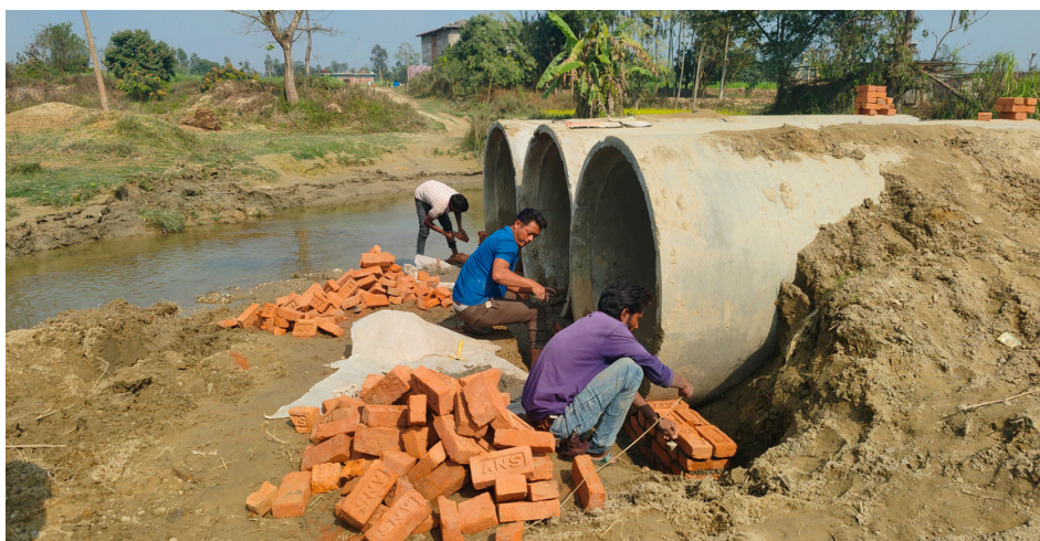
Culvert construction in Gujara Municipality of Rautahat district. Photo: RDC Nepal
