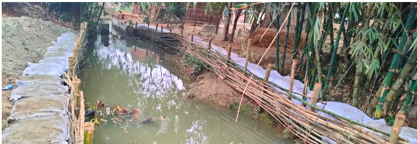
Construction of bio-embankment along Hardiya River. Photo: RDC Nepal
