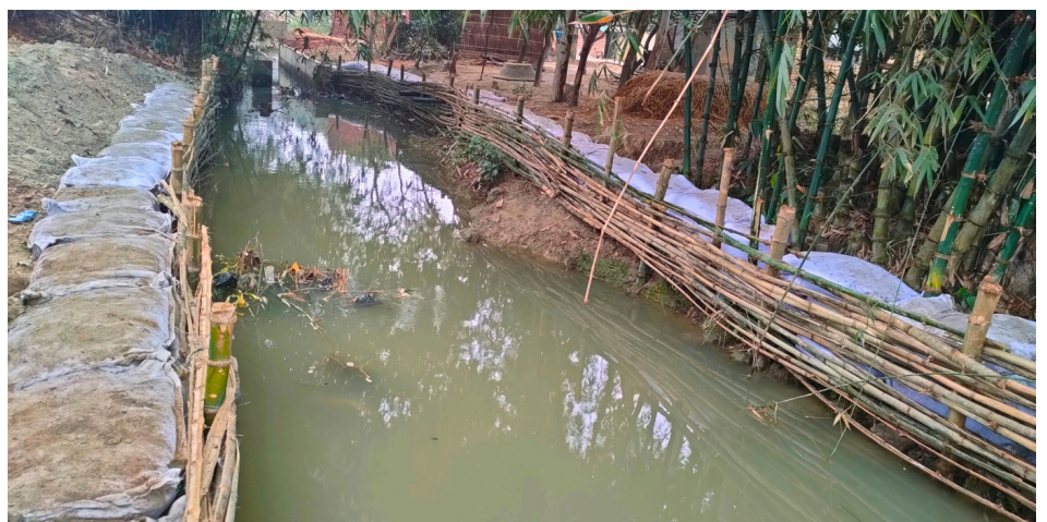
Construction of bio-embankment along Hardiya River. Photo: RDC Nepal
