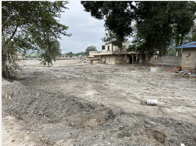
Destroyed Trishuli/Betrawati commercial area. Photo: Santosh Shrestha/Oxfam
