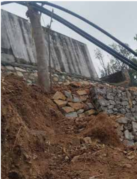
The reservoir tank of Kunekharka WSS on the verge of collapse due to the landslide. The landslide took away the earthen foundation across the edge of the reservoir.
