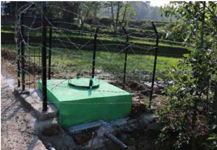
An interruption chamber chamber constructed under Bhakundebesi WSS to maintain water pressure
