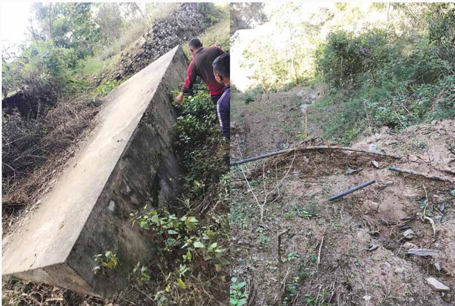
The landslide completely destroyed the reservoir tank and distribution pipelines, and the area was also covered in debris.
