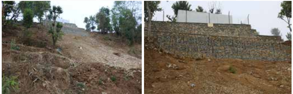
The repaired water reservoir with the protection wall under Kunekharka Water Supply and Sanitation Scheme (WSS). The structure was buried and damaged in mud by the landslide.
