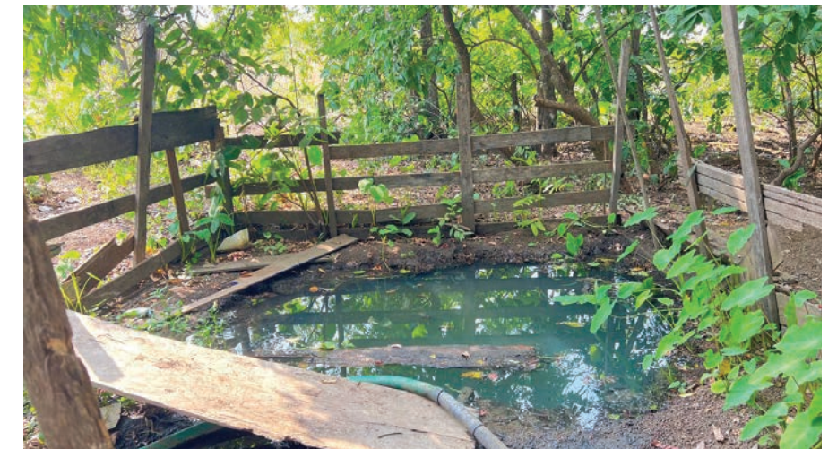
The water hole used by Chak Chap villagers before the bore wells installation. ©3SPN
